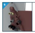
After about 2 minutes the protruding foam residue can be cut off with a suitable knife.
